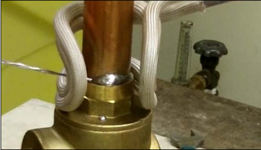
The assembly inside the induction heating coil during soldering
