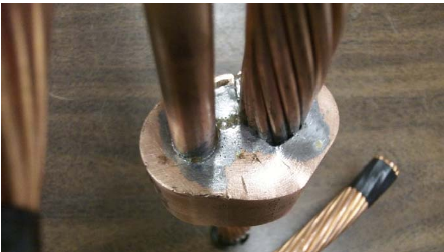
The joint made during the vertical orientation.
